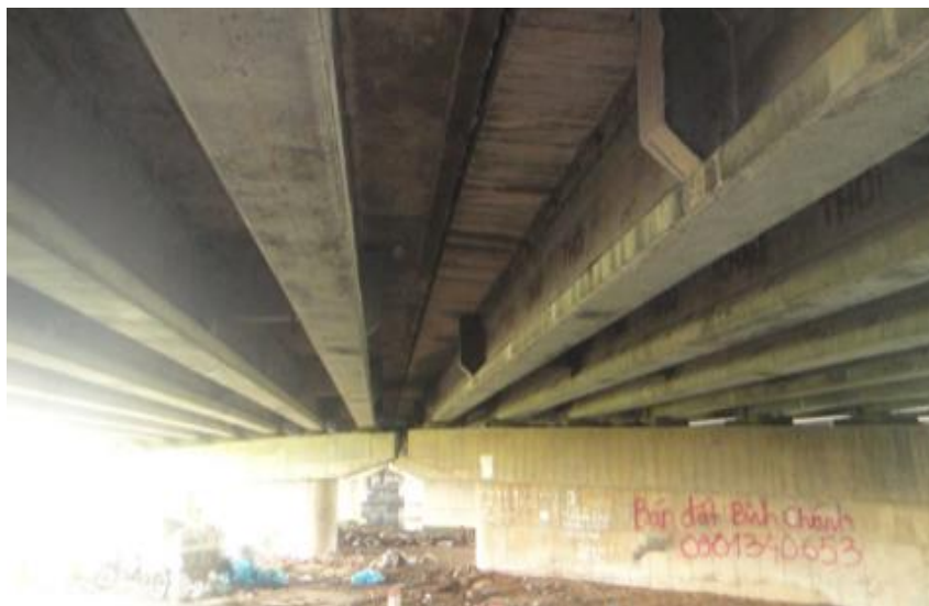
Figure 3. Measuring at the midpoint of the 19 th span.
