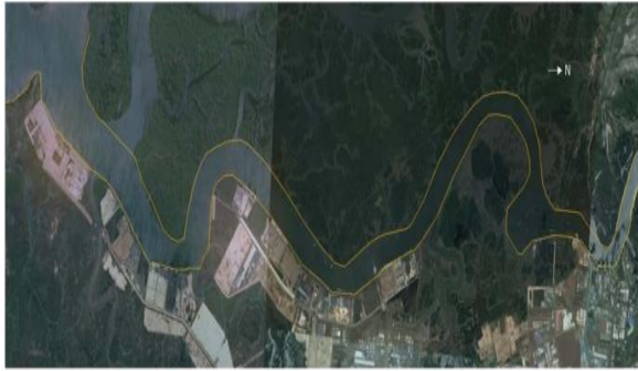
Figure 1. Overview of the Cai Mep-Thi Vai channel.
